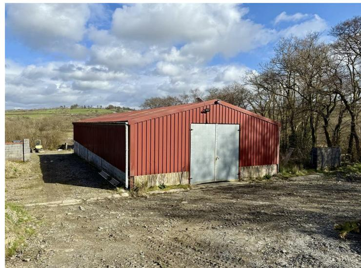
A useful modern portal framed barn with large opening doors to front and rear. This has been divided into 10 block built and rendered stable boxes, central bay, 4 other loose boxes and double doors on both ends.
